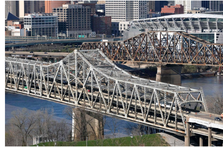
Brent-Spence Bridge (OH/KY)
