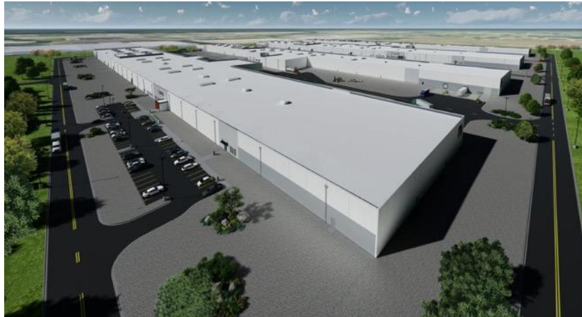
Illustration of ENTEK giga-scale factory in Terre Haute. Image sourced from ENTEK.
