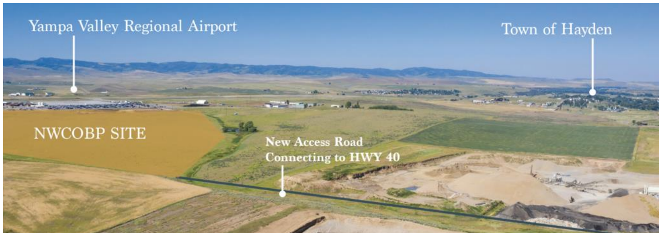
Aerial view of Hayden regional industrial park and surrounding area. Image sourced from Haydencolorado.com.
